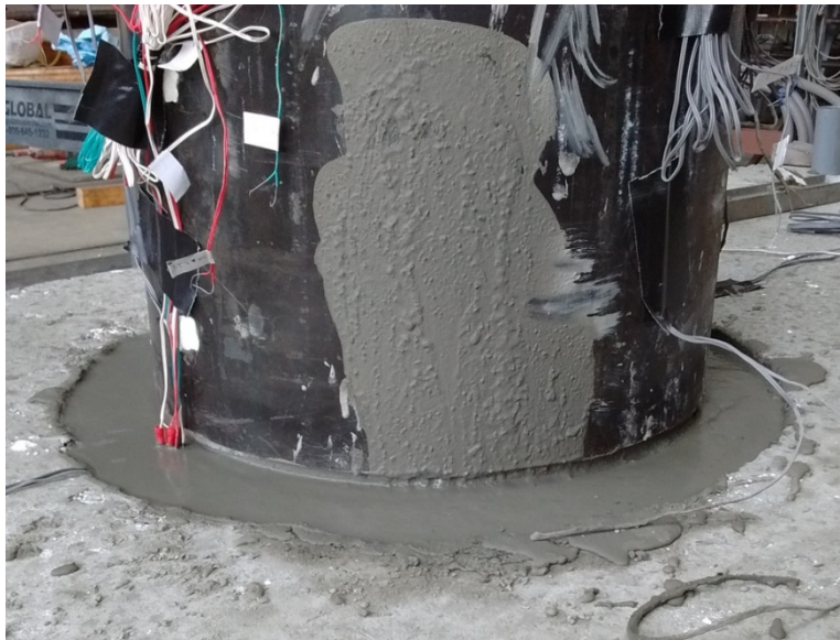
Figure 4.7 Grouting of columns in foundation socket.
