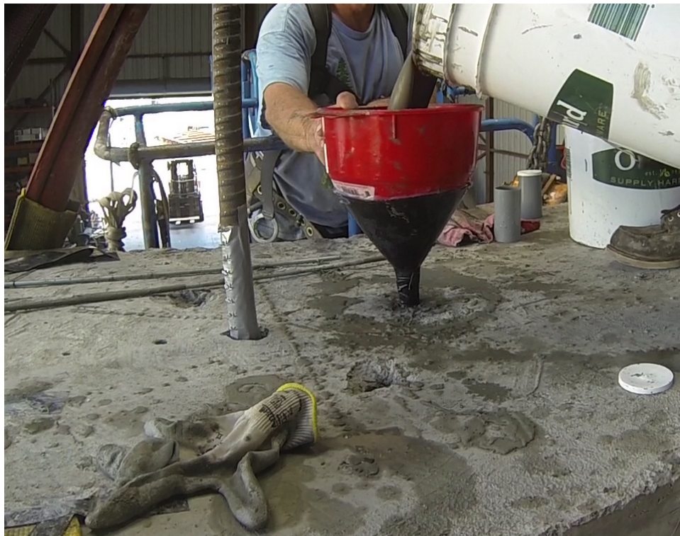
Figure 4.10 Grouting bent cap socket.
