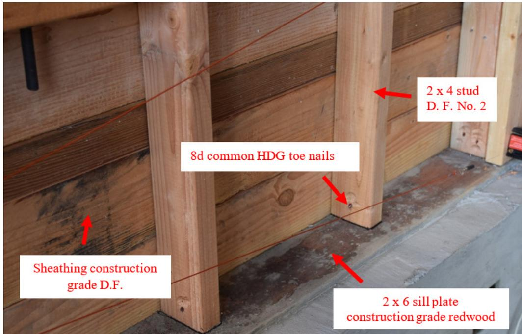
**Figure 3.24 Specimen A-6 wet set sill plate.**
