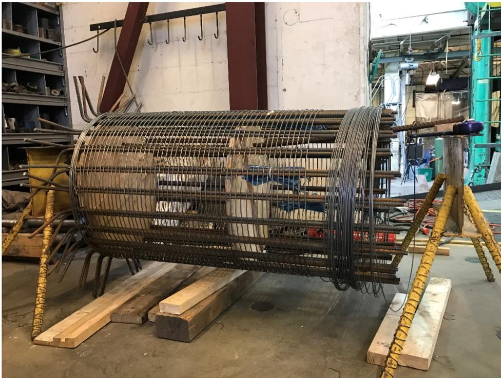
Figure B.1 Shaft reinforcement cage in progress.
