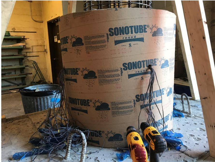
**Figure B.4** Sonotube formwork for the shaft, with strain gauge leads routed out.
