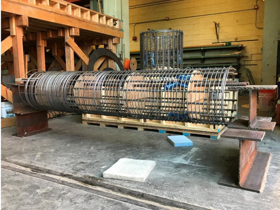
**Figure B.2** Column reinforcement cage in progress.
