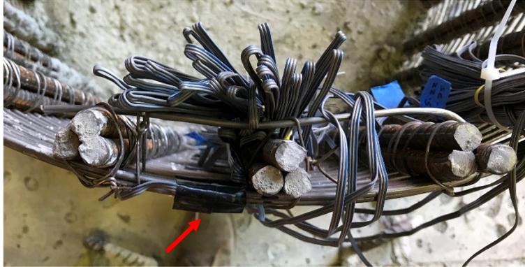
**Figure 5.18** Overhead view of uppermost wire strain gauge on the south end of the shaft reinforcement cage (indicated by red arrow; photograph was taken mid-installation).
