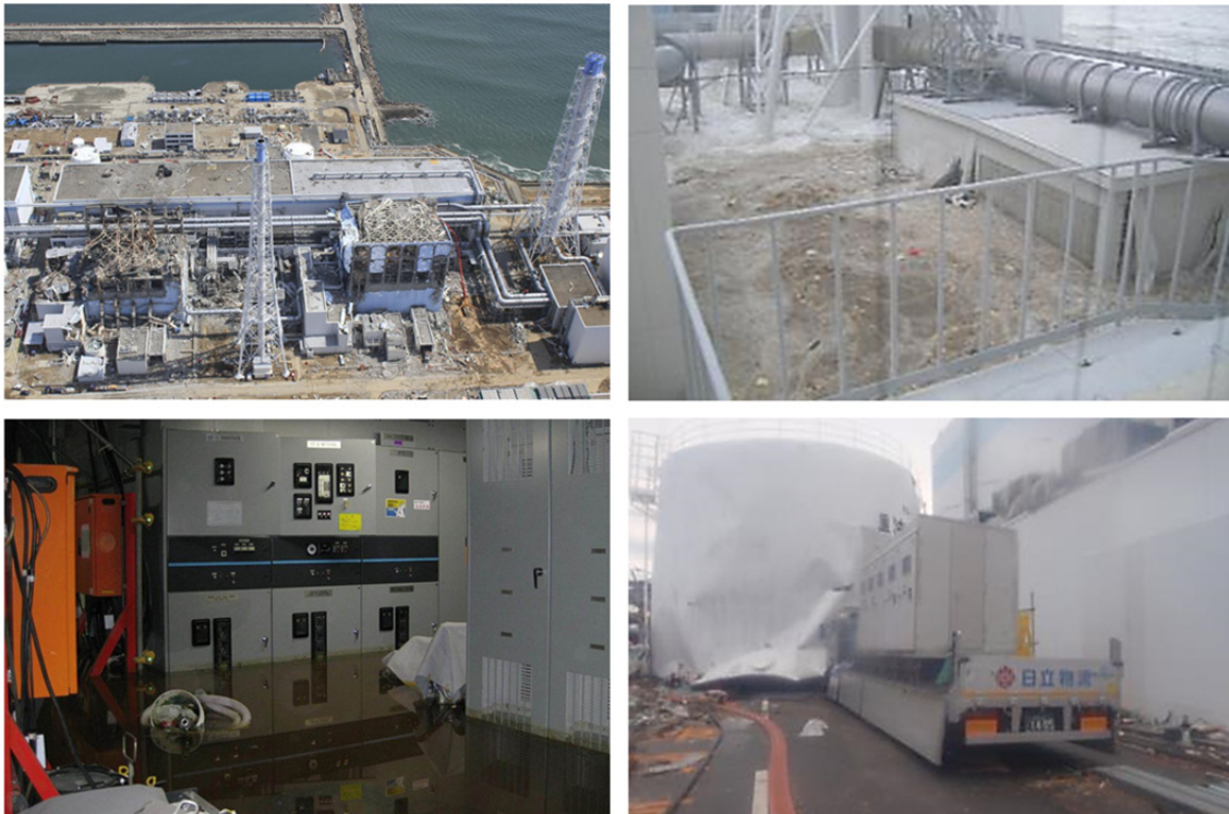
Figure 8.28 Photographs of the Fukushima nuclear power plant after the 2011 Tōhoku earthquake and tsunami.
