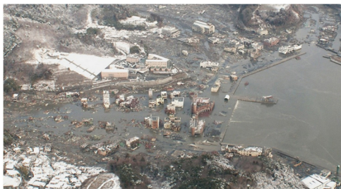
2004 Indian Ocean Tsunami Damage
