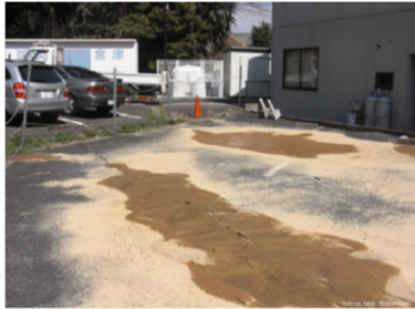
Sand ejecta observed in lower parking lot
