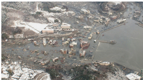
2004 Indian Ocean Tsunami Damage
