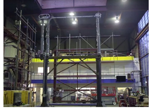
Disconnect Switch Testing
