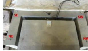
Bridge Seat Instrumentation
