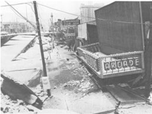
Figure 1.1 The head of the Fourth Avenue landslide induced by the 1964 Great Alaska Earthquake (Hansen 1965).
