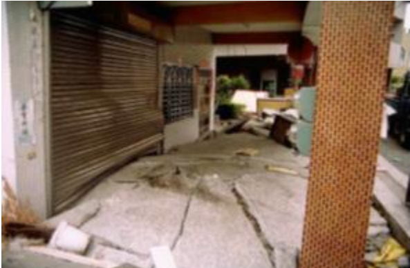
Figure 1.2 Typical foundation failure (punched footings and intermediate slab heaving). (Chu et al. 2008). Photo by R. Seed (1999)
