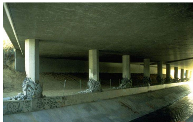
Plastic Hinge Damage
