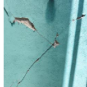
Shear damage
