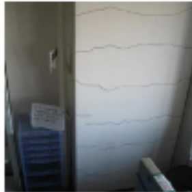
Flexural damage
