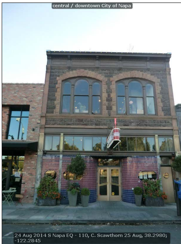
Figure 16 (t) block of URM buildings on Main Street Napa with little to no damage; (b) restaurant building in interior of the block in upper photo, retrofitted URM with no damage – note heavy steel columns also serving as wall bracing on interior.
