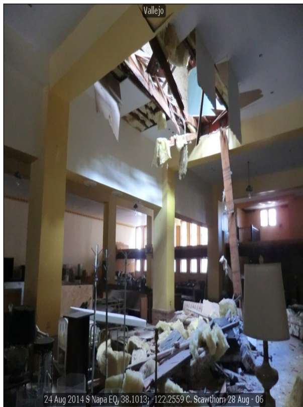
Figure 19 URM building, Georgia Street, Vallejo, (t) façade, with little apparent damage, note unbroken windows; (b) interior, showing ground floor on left and second floor on right, where parapet fell through to ground floor.
