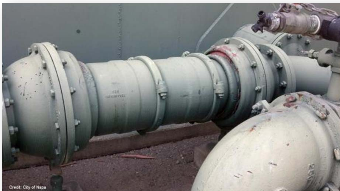
Figure 29 Montana “B” tank – roof damaged by sloshing and outtake exhibiting evidence of motion at slip joint.
