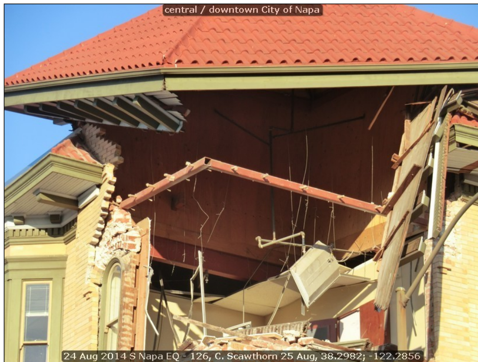
Figure 17 Heavily damaged URM building, Main Street Napa – note light horizontal member used in retrofitting, with clean pull out of masonry anchors.
