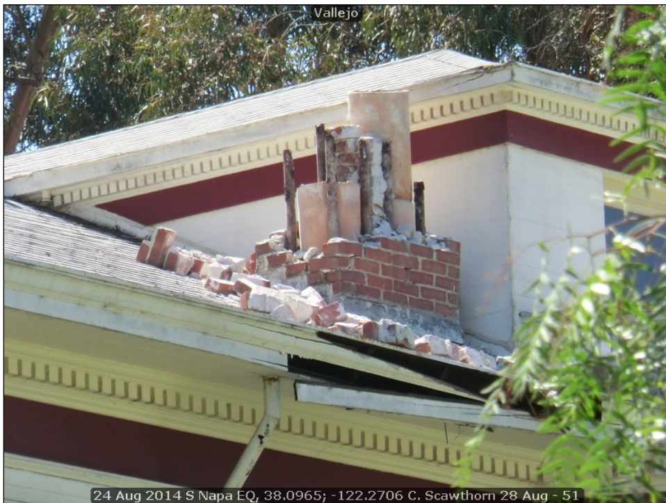
Figure 11 Approximately 1900 era house with chimney damage, Mare Island
