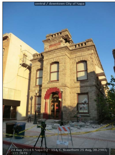
Figure 21 Goodman library – URM built 1901, longest continuously operating library in California, National Register #74000539, retrofit unclear, damaged.
