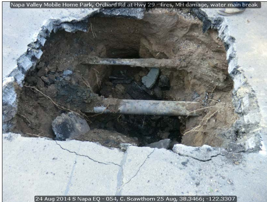
Figure 27 Water main break, Orchard Road.
