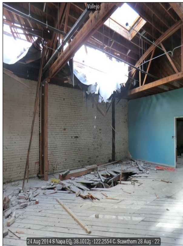
Figure 19 URM building, Georgia Street, Vallejo, (t) façade, with little apparent damage, note unbroken windows; (b) interior, showing ground floor on left and second floor on right, where parapet fell through to ground floor.
