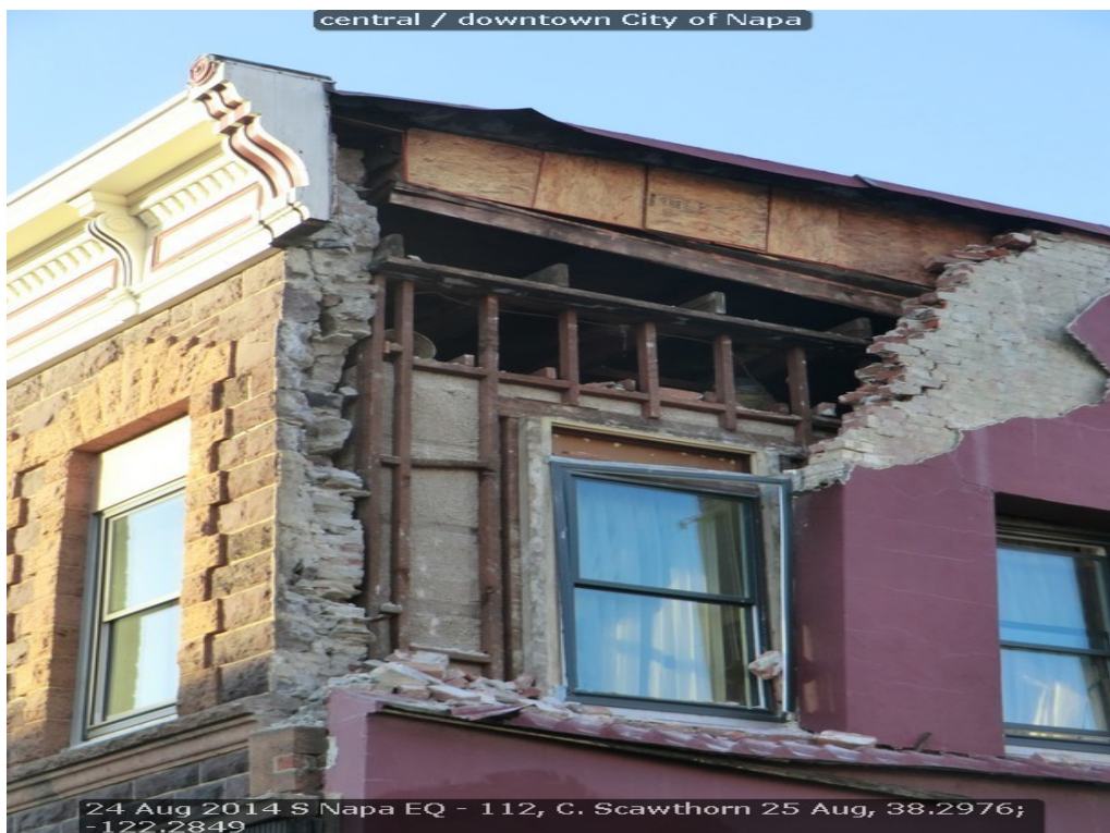
Figure 18 Building directly across Main Street from buildings in Figure 16 with no apparent retrofitting and partial loss of second story wall.
