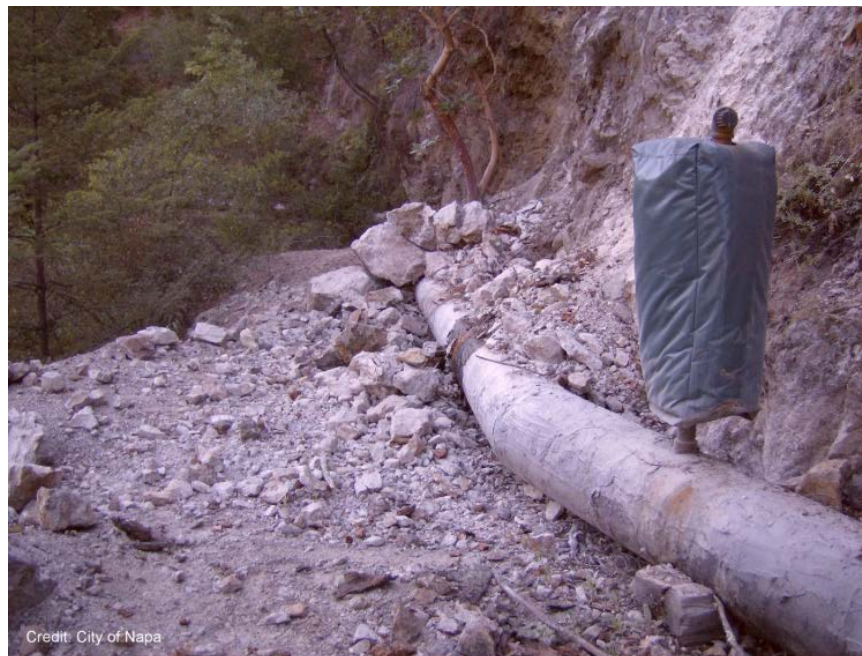
Figure 28 Milliken line, broken by rock slide.
