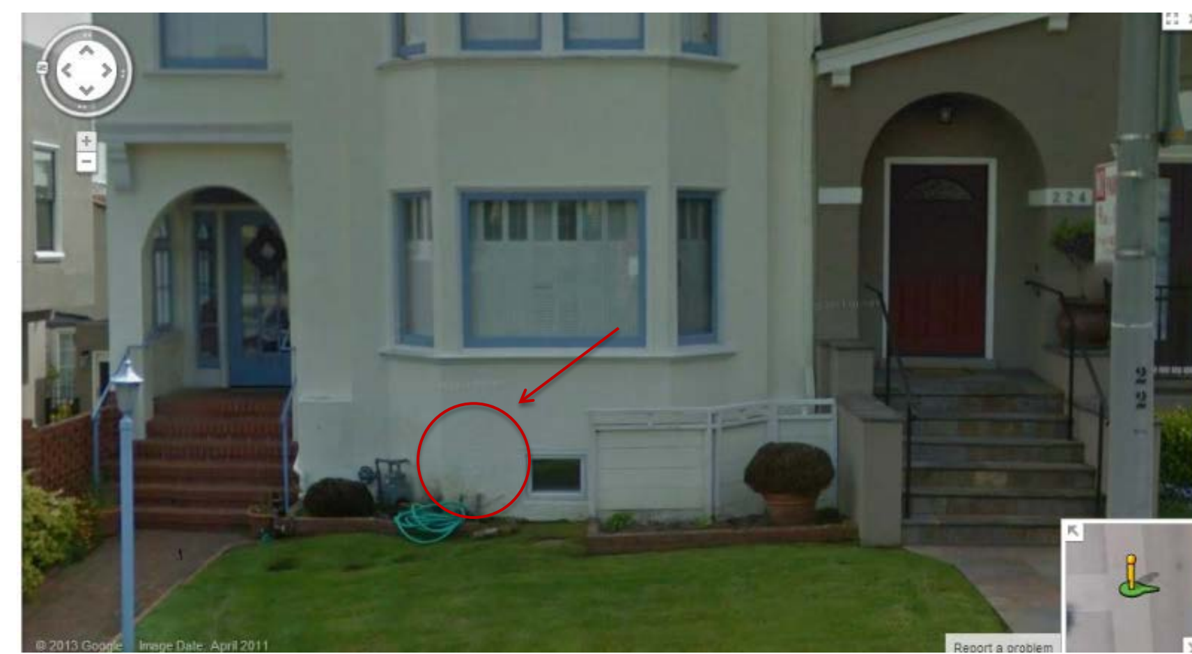
Figure 3. Front view of a home with cripple wall. Hints include vent and the number of steps (Google)
