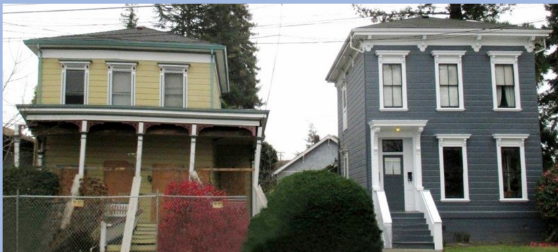
Figure 10. A two-story house with wood siding (LEFT) was heavily damaged and unusable after the 2014 South Napa, CA earthquake while a similar retrofitted one (RIGHT) remained occupied. – Photo credit: CEA
