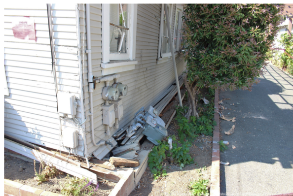
Figure 2. The unbraced crawlspace walls of this wood-frame house racked and collapsed, breaking utility connections and leading to a red tag designation in the 2014 South Napa, CA earthquake. – Photo credit: Petros Keshishian
