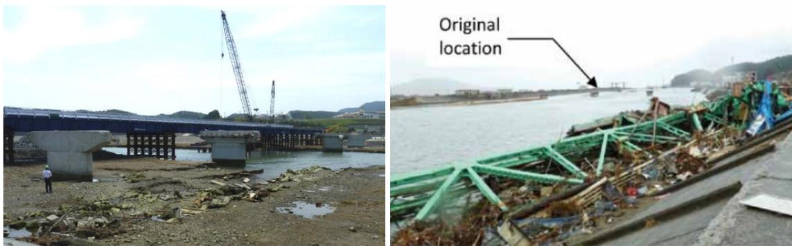
**Figure 1.1: Damaged bridges after the 2011 tsunami in Japan: (a) Koizumi bridge on the left (source: EERI Oct. 2011) and (b) Bridge in Rikuzentakata on the right (source: EERI Sept. 2011)**
