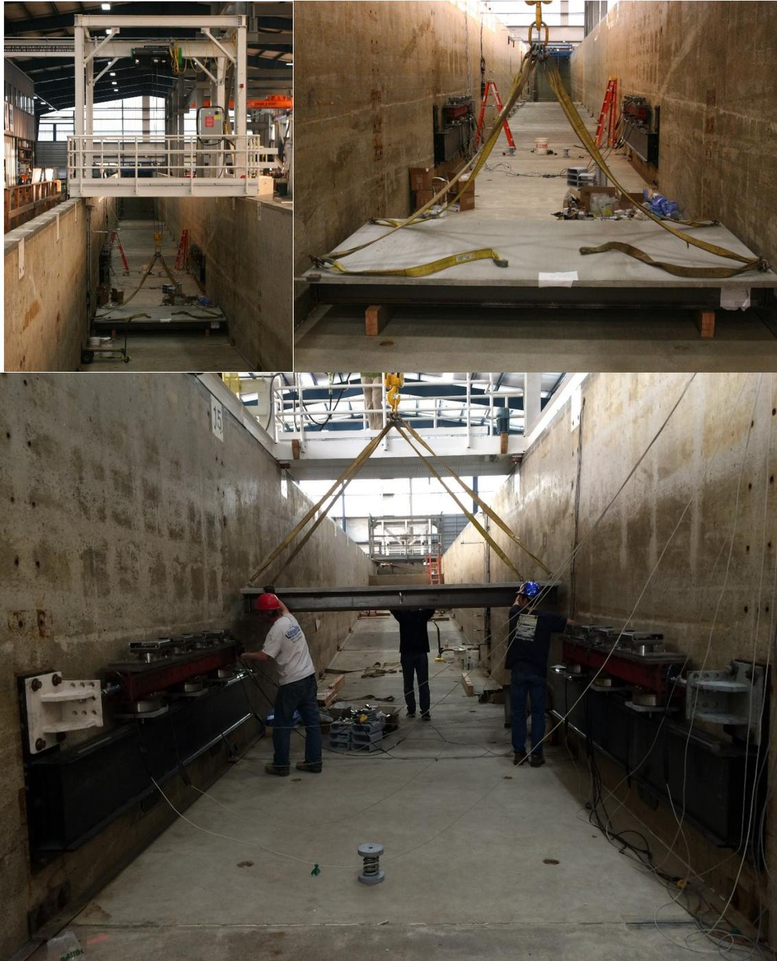
**Figure 1.14: Installation of the bridge with steel bearings in the LWF**
