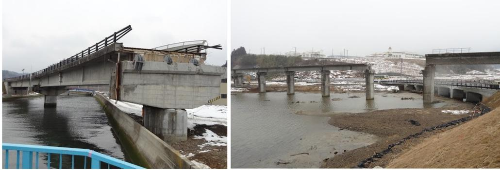
**Figure 1.2: Damaged bridges after the 2011 tsunami in Japan: (a) Utatsu bridge on the left and (b) Tsuya railway bridge on the right (adapted from Yashinski, M 2012)**
