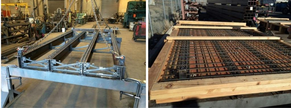
**Figure 1.4: Bridge steel components during the assembly (left) and before the concrete pouring (right)**
