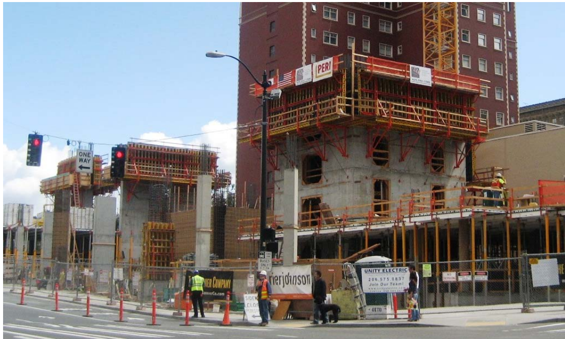
Figure A-3 Construction of concrete walls for a high-rise apartment building. The structural system has two individual walls, at left, and a concrete core, at right (courtesy of KPFF).
