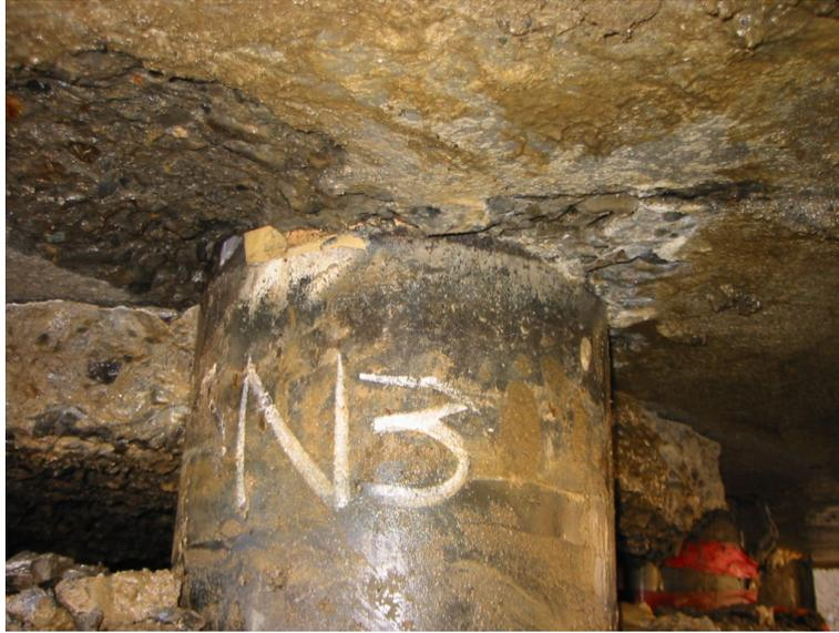
**Fig. 5.29 Concrete spalling underneath pile cap of 4-pile group (pile N3)**
