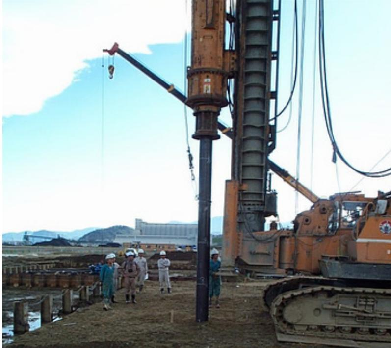
**Fig. 4.8 Pile driving using diesel hammer**
