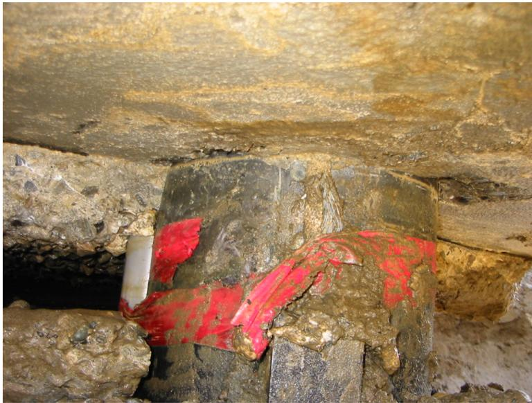
**Fig. 5.30 Concrete spalling underneath pile cap of 9-pile group (pile No. 8)**
