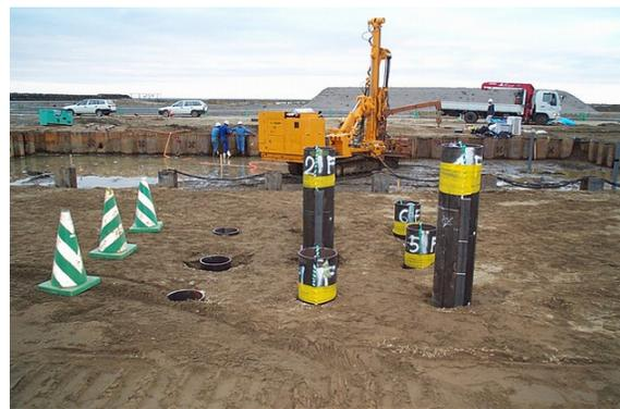
**Fig. 4.9 Pile length left over after pile installation: (a) 4-pile group (left), (b) 9-pile group (right)**
