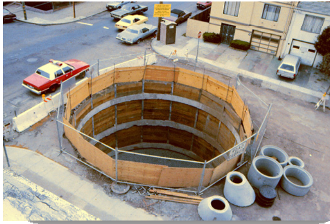
Figure 3.5 Typical San Francisco Fire Department cistern under construction.
