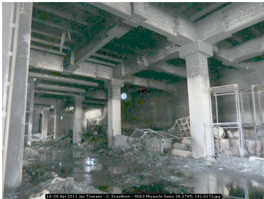
Figure 2.22 Interior of warehouse above, 2011 Eastern Japan earthquake (courtesy of C. Scawthorn).
