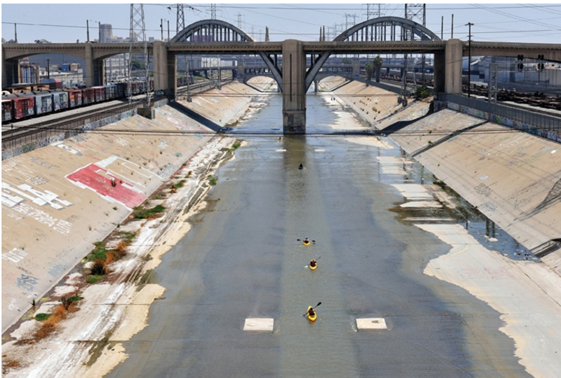
Figure 4.4 Los Angeles: one of the larger storm drain channels.
