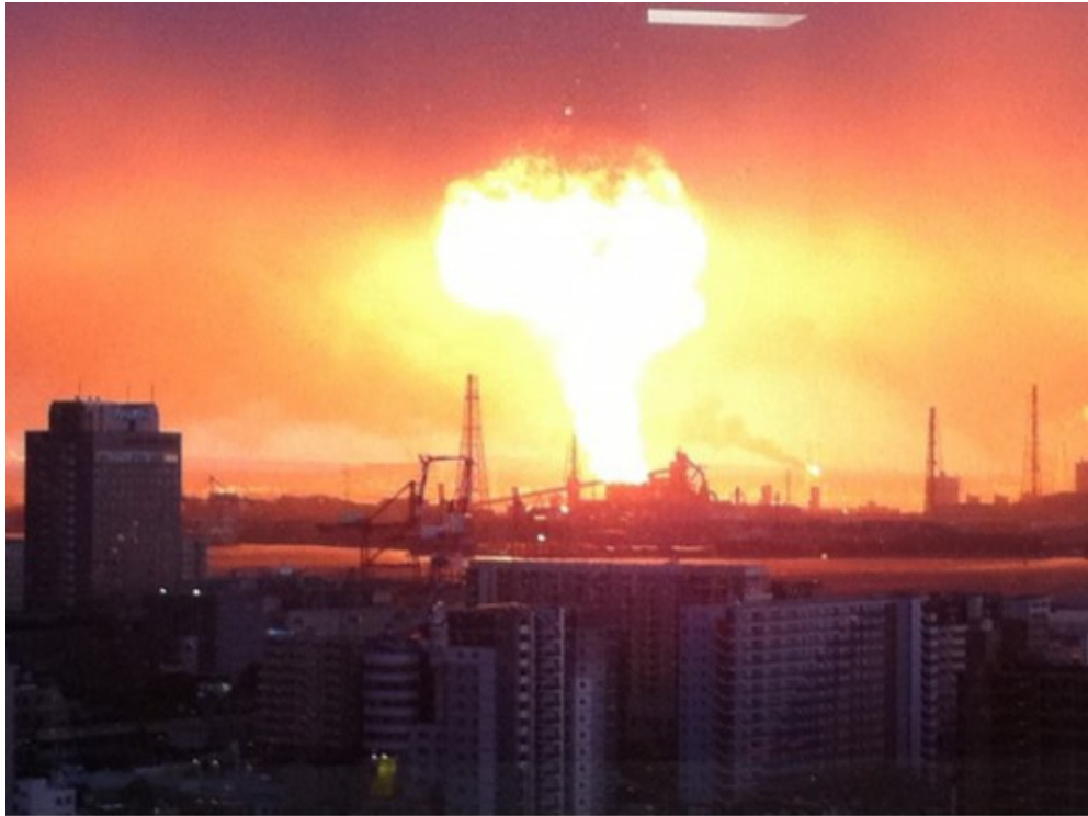
Figure 2.18 Gas sphere ignition at Cosmo Refinery, Chiba, 2011 Eastern Japan earthquake (courtesy of www.planetsave.com ).
