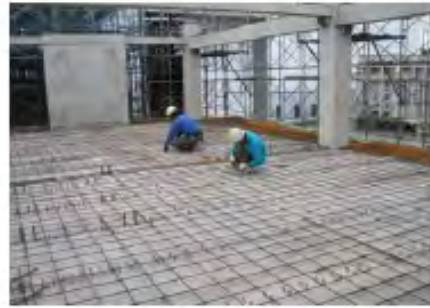
(e) Steel arrangement for top slab
