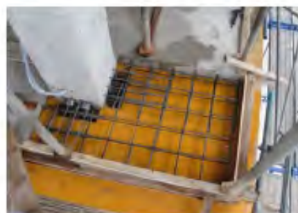
(h) Steel arrangement for corner slab
