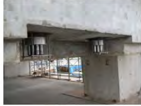
(f) Anchorage of PT wires beneath foundation
