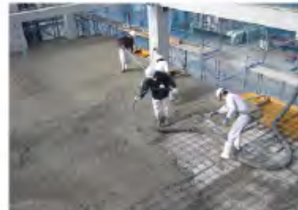
(f) Cast of top concrete
