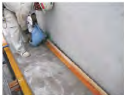
(h) Fiber mortar for wall bed
