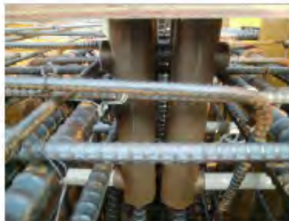
(b) Couplers for energy dissipating element (D22)
