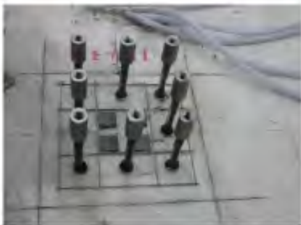
(c) Threaded couplers above foundation
