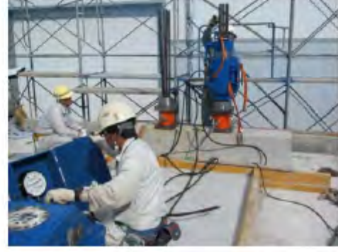
(g) Pump and jack prestressing PT wire
