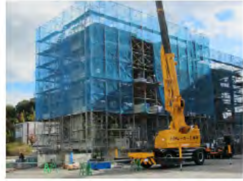
(e) Preparation for prestressing the multi-story wall
