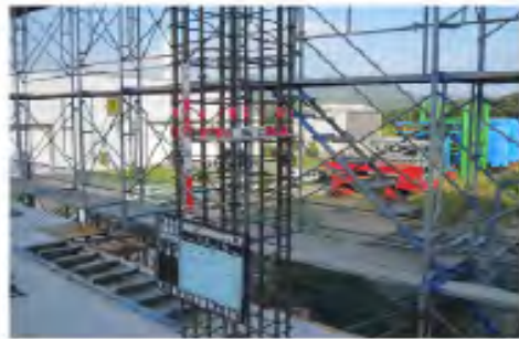
(c) Steel arrangement of column
