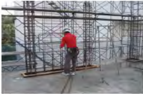
(b) Steel arrangement of wall
