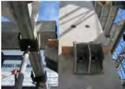
(b) Bracket supporting beam end
