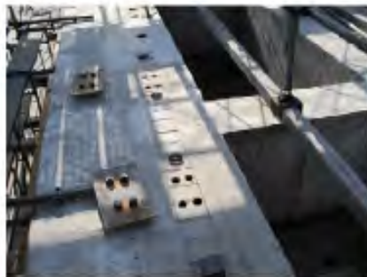
(c) Foundation before wall-set (holes for PT wires and D22)
