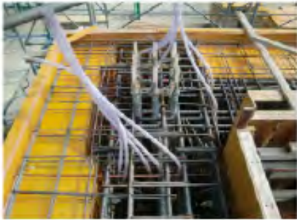
(b) Steel arrangement of foundation
