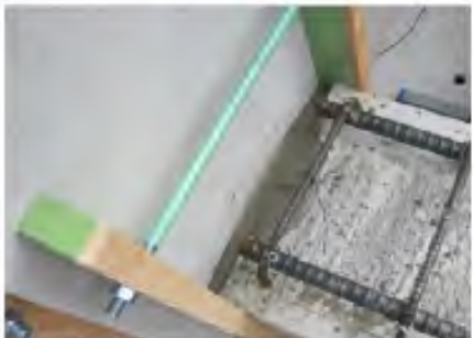
(c) Grouted beam end (mortar)
