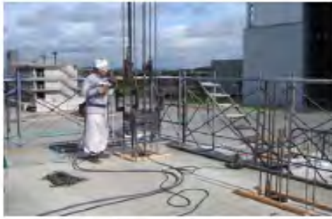
(a) Gas pressure welding
