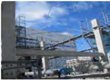
(a) Placing half precast concrete beam
