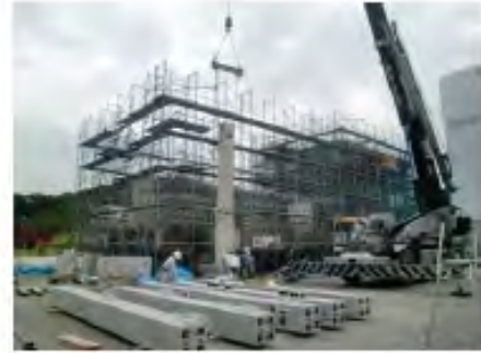
(e) Lift-up of the precast concrete column
