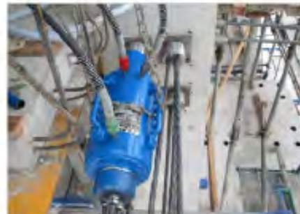
(g) Beam prestressed after concrete cast
