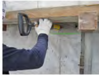
(e) Grouted coupler (injection of mortar)
