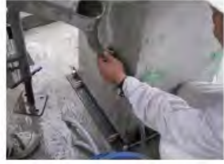
(g) Grouted column bed (mortar)
