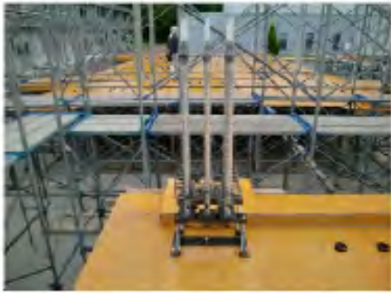
(a) Anchorage of PT bars in foundation
