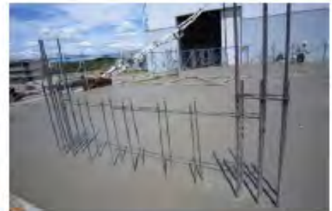
(g) Concrete cast
