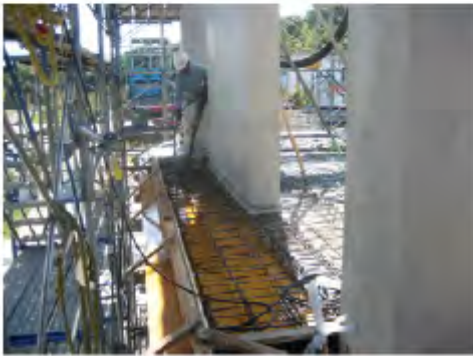
(c) Concrete cast around wall
