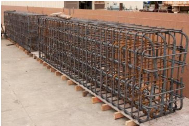
**Figure A.7** Assembled foundation reinforcing bar cages.
