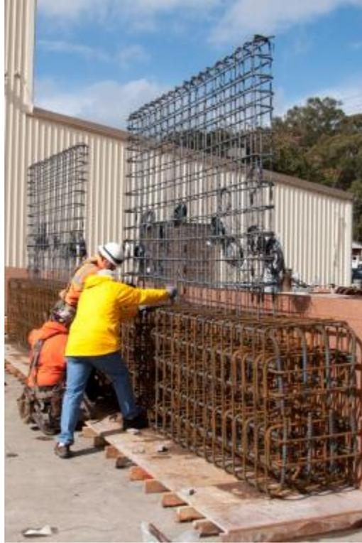
**Figure A.8 Wall and foundation reinforcement.**
