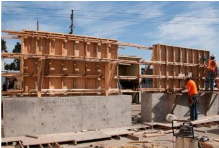
**Figure A.11** Walls formwork.
