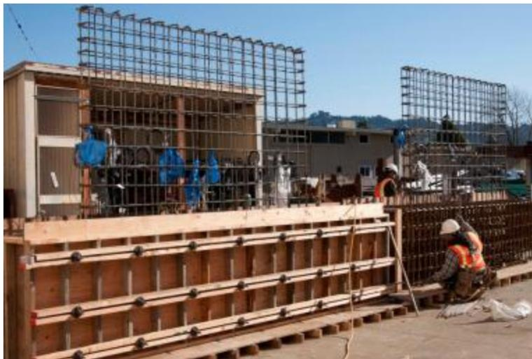
**Figure A.9 Building formwork.**
