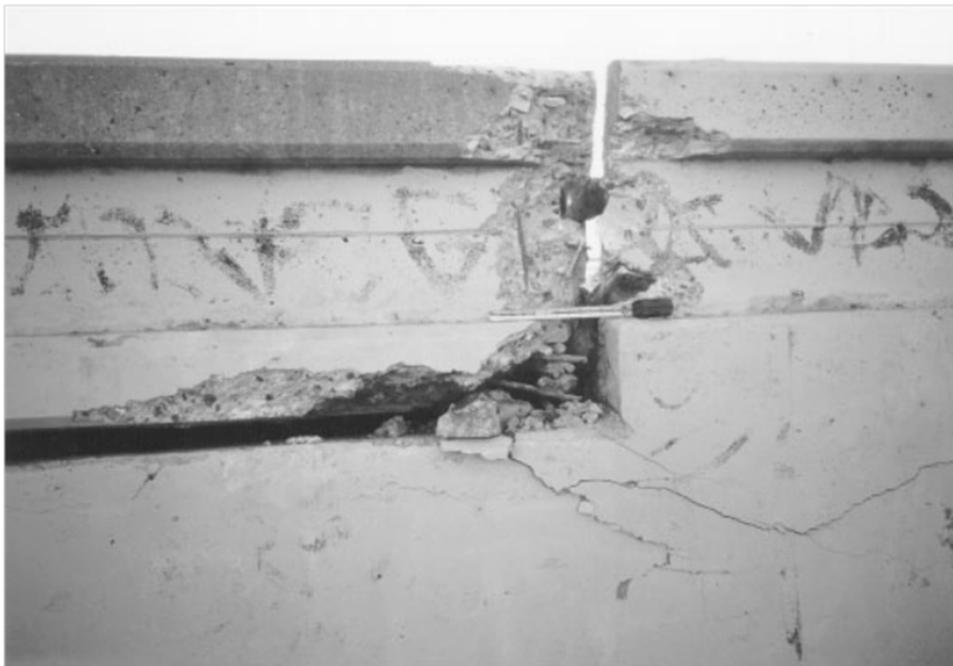
**Figure 1.3** Santa Clara River Bridge pounding damage to the abutment in 1994 Northridge Earthquake (source: Chen and Duan [2000]).
