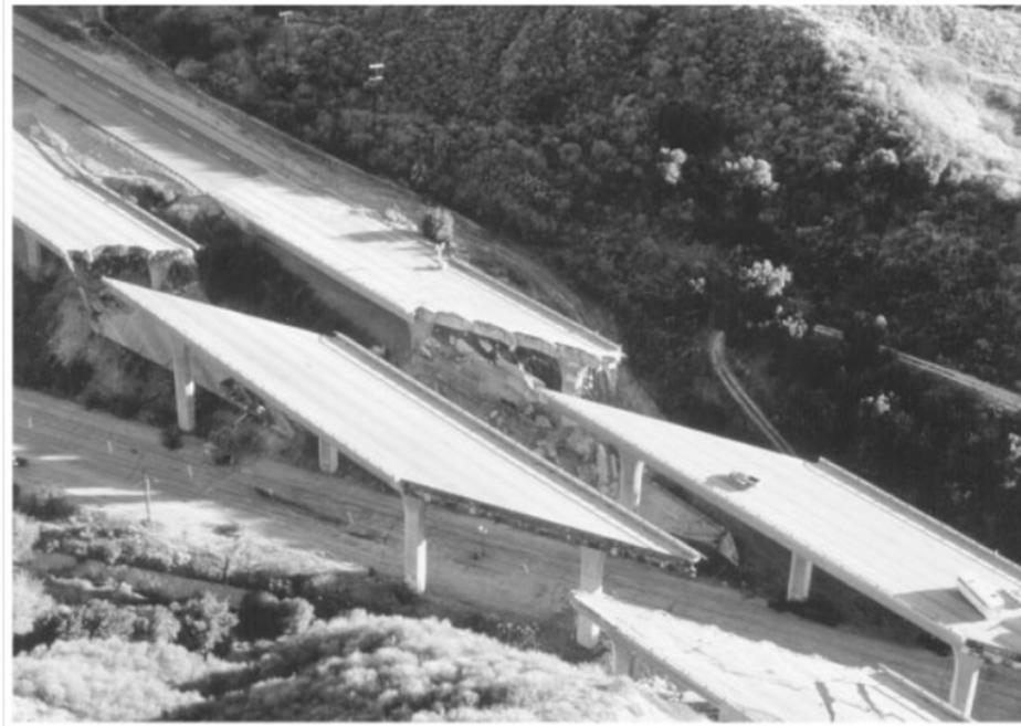
**Figure 1.2** Gavin Canyon Undercrossing collapse in the 1994 Northridge Earthquake (source: Chen and Duan [2000]).
