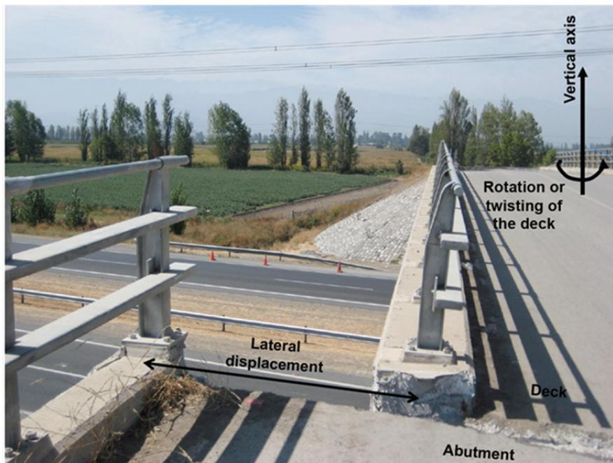
Figure 1.5 Damage to a skewed bridge after the Chile Earthquake of February 27, 2010 (source: Yashinsky et al. [2010]).
