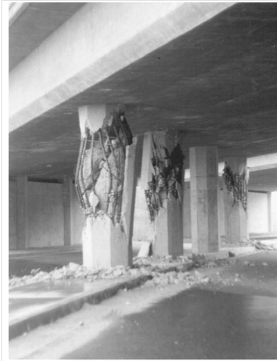
**Figure 1.1** Failure of columns of the FBU (source: Chen and Duan [2000]).
