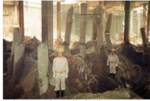
Pile damage in soil during 1964 Niigata; damage disclosed after twenty years during renovation.
