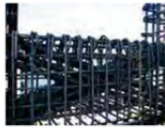
Conventional diagonally reinforced coupling beams
