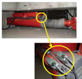
2 stage variable-orifice damper
