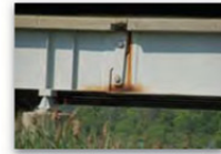
Link plate and pin assembly
