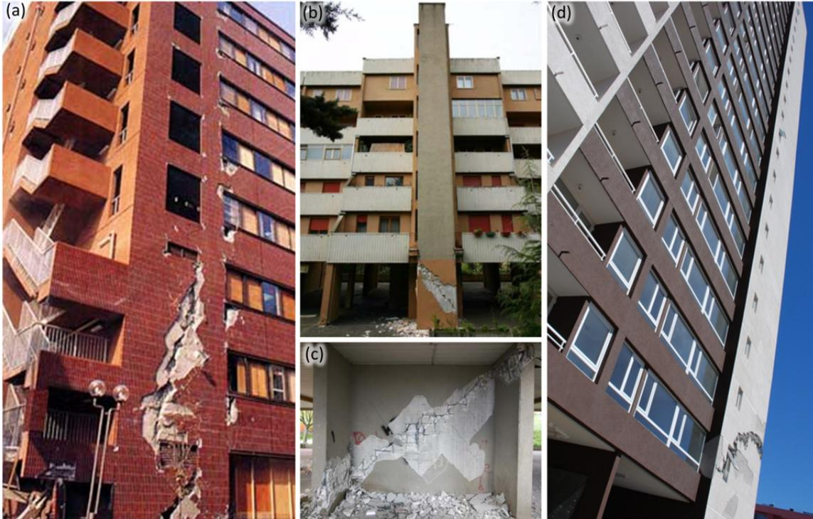
**Figure 1.1** Photographs of diagonal tension and compression failures taken after major earthquake events: (a) M6.8 1995 Kobe, Japan earthquake (from Maffei and Yuen [2007]); (b-c) M6.3 2009 L'Aquila, Italy earthquake (from Dazio [2009b]); and (d) M8.8 2010 Chile earthquake (courtesy of J. Restrepo).
