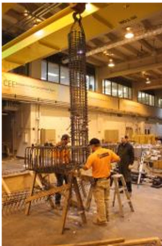
Figure C.5 Different stages of assembling the bent cap beam and column cages then installing the assembly in place using the overhead crane
