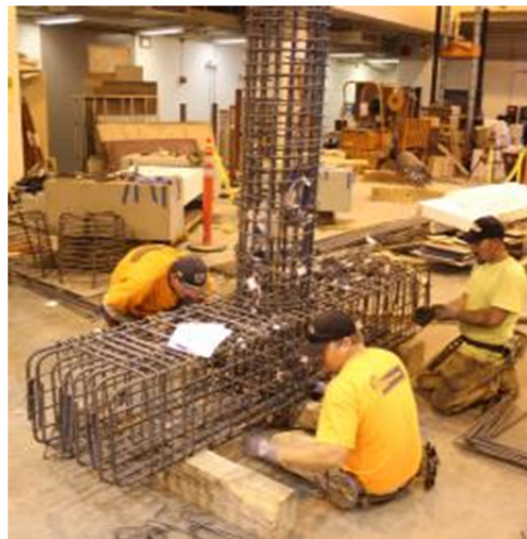
Figure C.5 Different stages of assembling the bent cap beam and column cages then installing the assembly in place using the overhead crane
