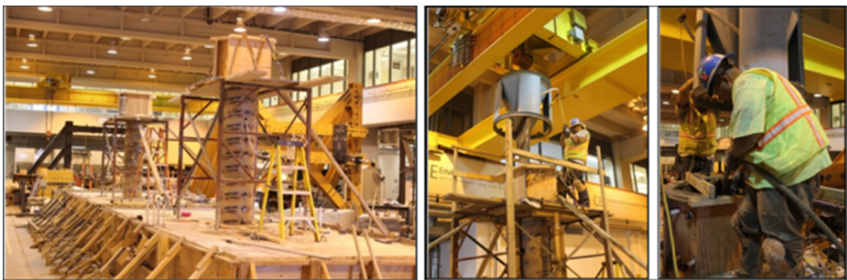
Figure 3.20 (a) Finishing the surface of the second concrete lift and (b) curing of concrete surface using curing blankets.
