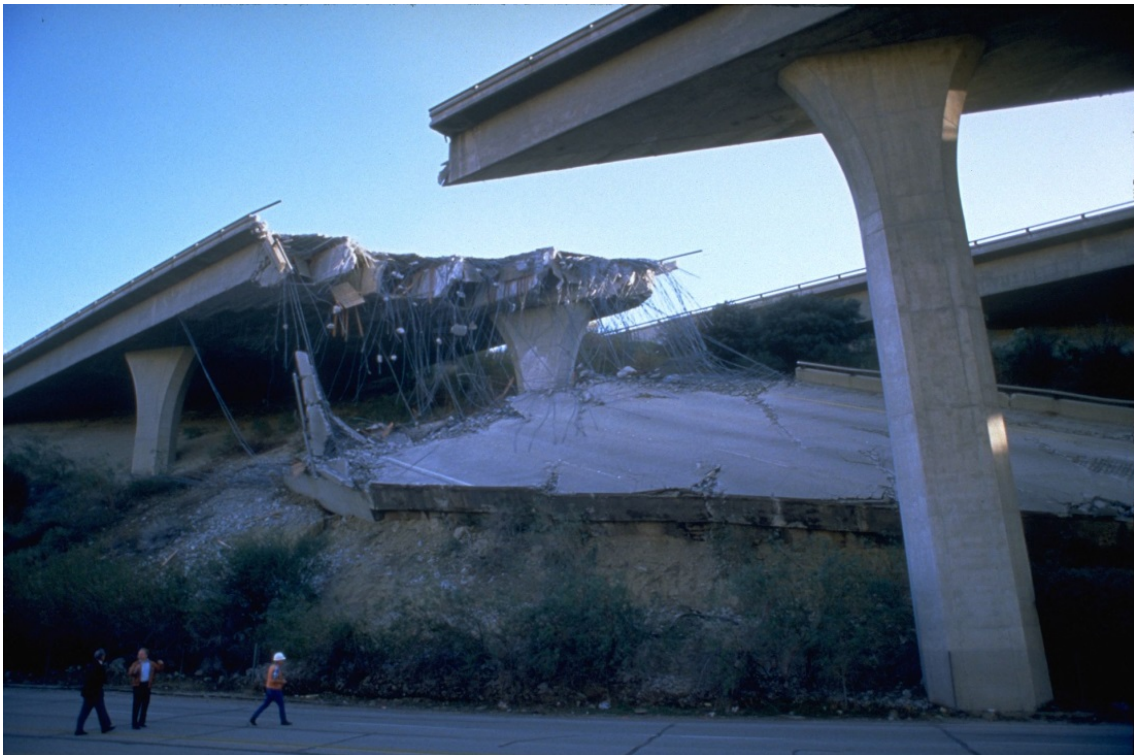
Figure 1.3 Damaged portion of the Golden State Freeway, part of CA Interstate-5, at Gavin Canyon after 1994 Northridge earthquake (courtesy of FEMA Photo Library).
