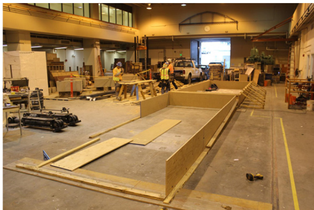
Figure C.1 Laying out the construction space and setting up the formwork for the seat beams of the specimens.
