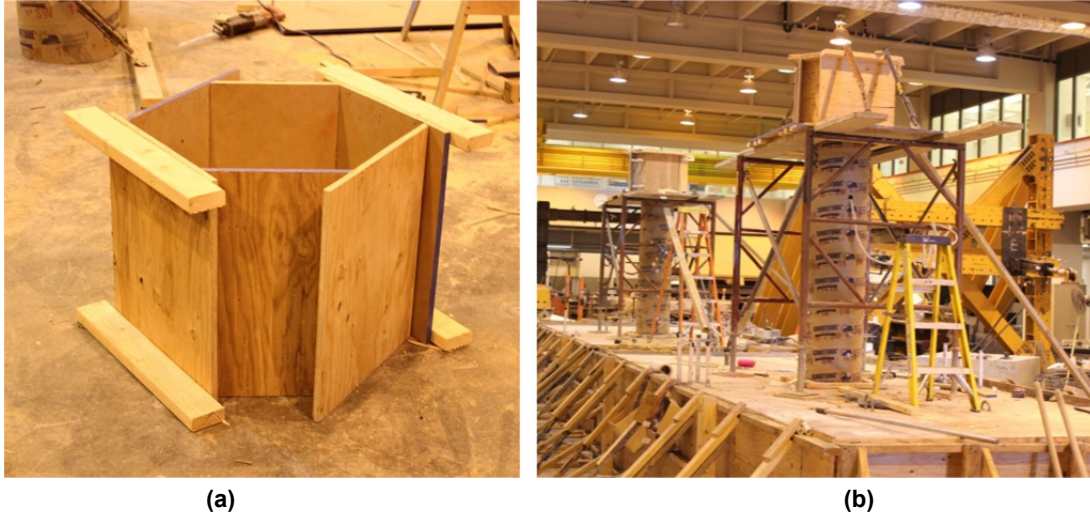
Figure C.12 (a) Special hexagonal formwork for the column head; and (b) overview of the complete formwork and scaffolding for the columns and column heads.
