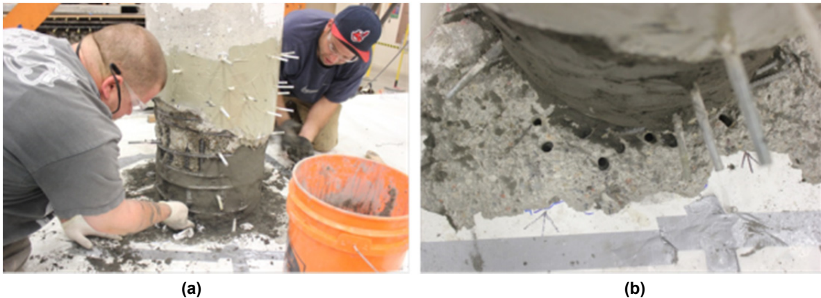
Figure 6.4 (a) Patching the column damaged core with high-strength mortar in the plastic hinge zone; and (b) 8-in.-deep vertical holes to add polymer reinforcing bars.
