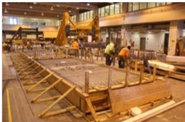
Figure C.2 (a) Preparing styrofoam blocks used to fill the void between seat beams, which were then covered with plastic; and (b) fabricating the reinforcement cage of the seat beams.
