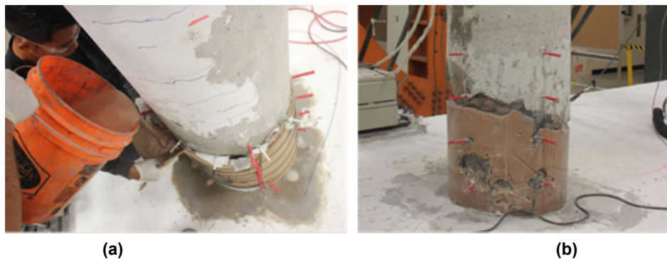
Figure 6.8 (a) Pouring sand-epoxy mixture inside the sonotube formwork to restore the column shape; and (b) view of the partially repaired column after the sonotube was removed.
