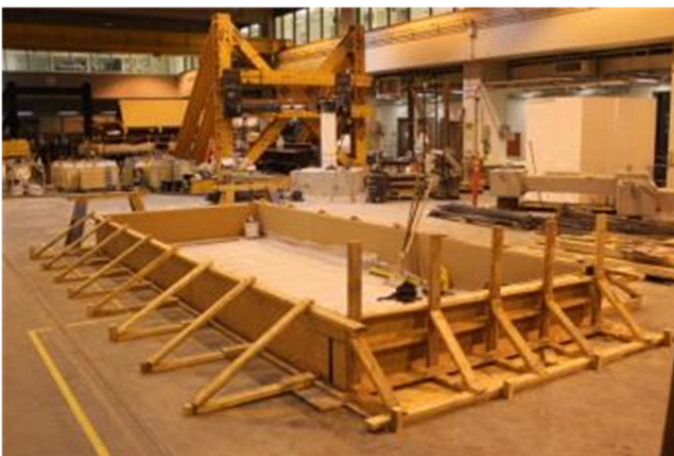
Figure C.1 Laying out the construction space and setting up the formwork for the seat beams of the specimens.
