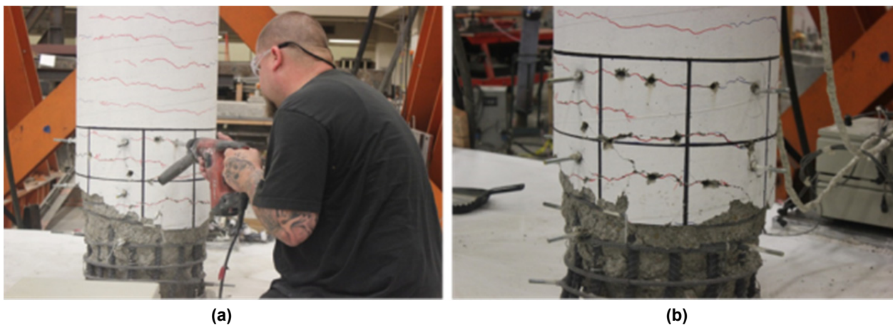
Figure 6.2 (a) Drilling holes along the cracks for epoxy injection; and (b) final pattern of injection sites for repair with epoxy.
