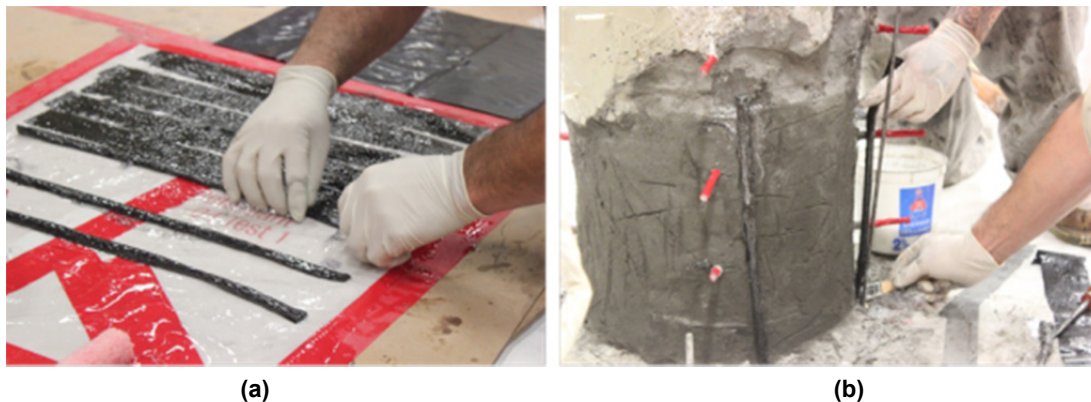
Figure 6.5 (a) Preparation of 20-in.-long CFRP bars using carbon fiber sheets coated with epoxy resin; (b) installing the wet CFRP bars in the holes drilled into the cap beam.
