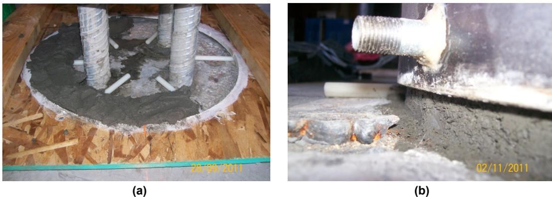
**Figure 3.5** Mortar bed: (a) wood template and nylon-rod shims, during mortar placement; and (b) mortar scraped from underneath the outer shell.
