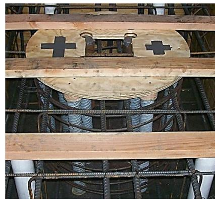
**Figure 3.3** Footing details: (a) horizontal section; (b) longitudinal section; (c) reinforcement, ducts, and formwork; and (d) steel ducts and spiral reinforcement.
