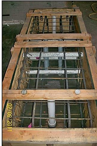
Figure 3.4 Load-stub details: (a) horizontal section; (b) longitudinal section; and (c) reinforcement, ducts, and formwork.
