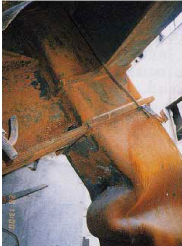
Figure 2.10 Local buckling at the top of a cold-formed square hollow section column in a 5-story moment-resisting steel frame [AIJ 1995].
