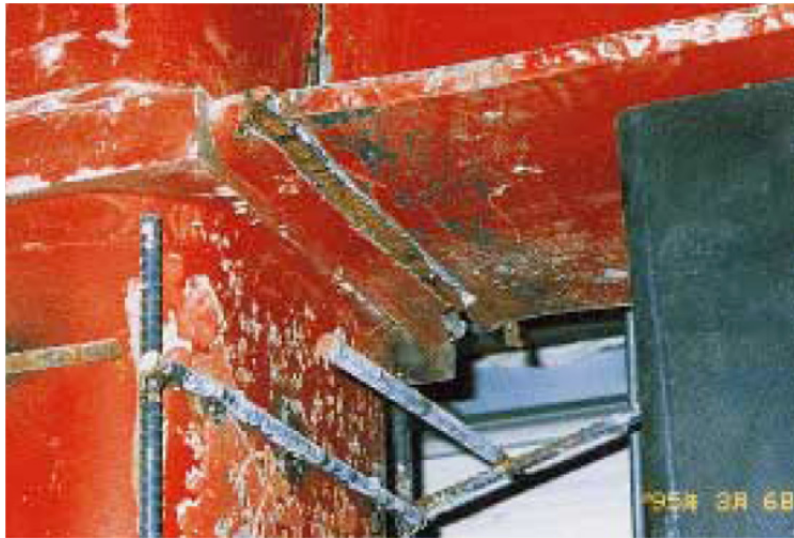
Figure 2.8 Beam bottom flange and partial web fractures in a 5-story moment frame [AIJ 1995].
