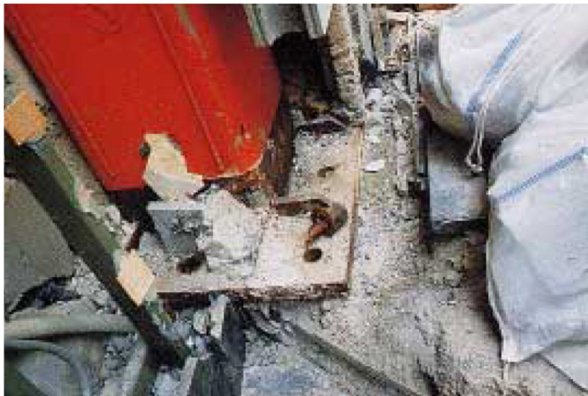
Figure 2.11 Fracture of anchor bolts and shifting of base plate in a 6-story steel moment-resisting frame [AIJ 1995].
