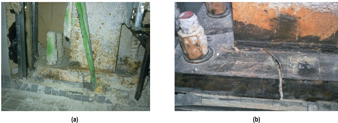
Figure 2.6 Steel column base plate damage observed at Oviatt Library; (a) overview of column base and (b) closed view of crack in the base plate (sources: NISEE and EERI [1997]).
