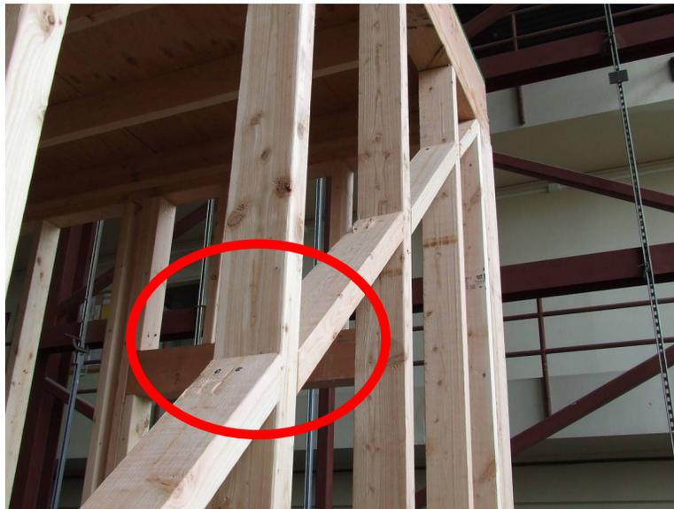
**Fig. 5.5 Blocking used to brace shear-wall framing of test structure B.**
