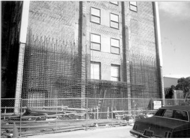
One of the main considerations driving the selection of the jacketing scheme was the need to keep Barrows Hall open during the construction process. The retrofit of Barrows was scheduled to begin in July of 2000 and to end in July of 2002. At the time, the university was already engaged in several retrofit projects and there was not enough surge space to accommodate the faculty, staff, and students that occupied Barrows Hall.
