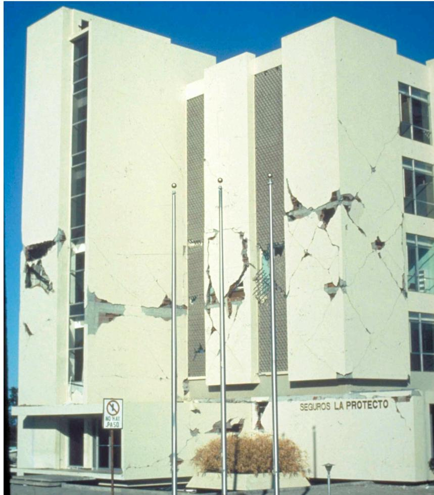
**Fig. 8.13** Five-story RC building with URM infill walls damaged during magnitude 6.19 Nicaragua earthquake, 12/23/1972. (Courtesy Godden Collection, EERC, University of California, Berkeley.)
