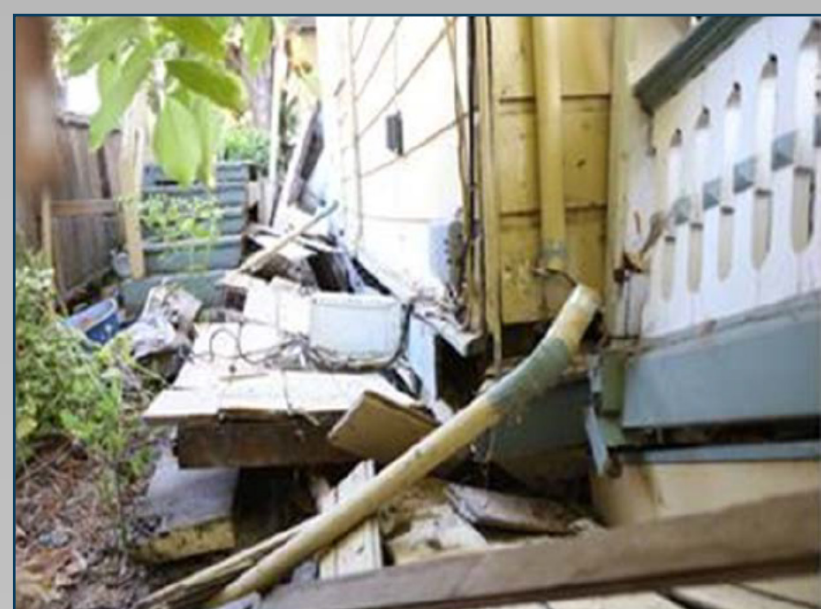
Cripple wall failure (2014 South Napa)
