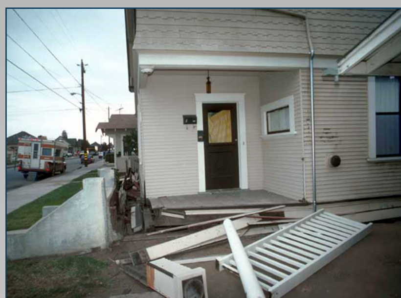
Cripple wall failure (1989 Loma Prieta)
