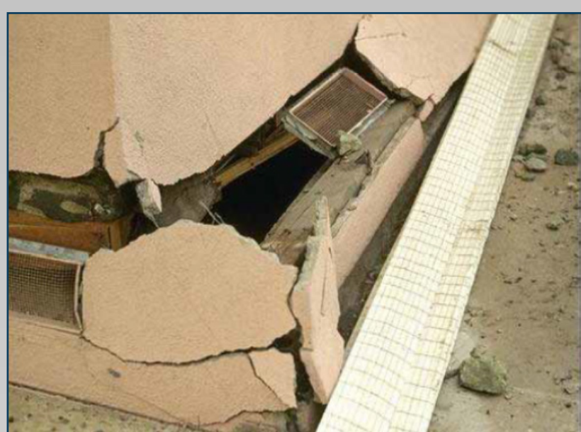
Sill anchorage failure (1971 San Fernando)
