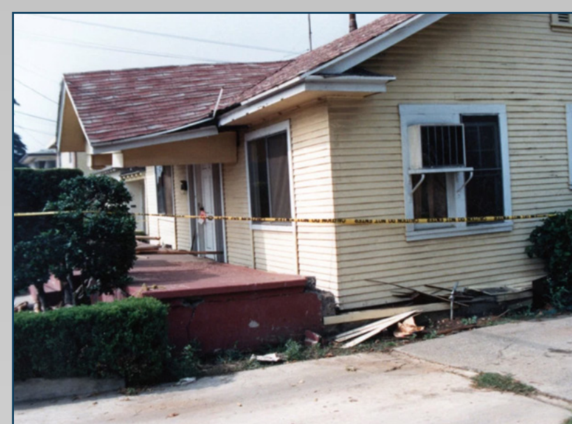
Cripple wall failure (1987 Whittier Narrows)
